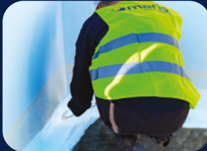
STEP 5 Wall-floor connection
