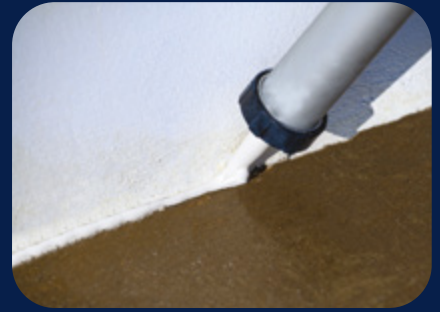
STEP 3 Fixing cracks and joints
