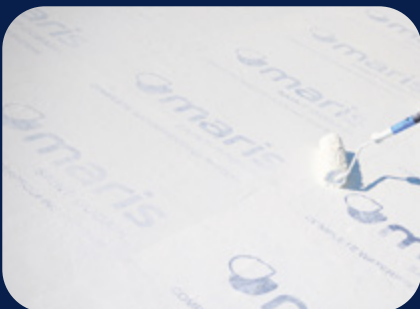
STEP 7 2nd layer of waterproofing membrane
