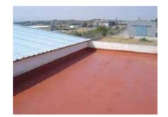
After curing of the waterproofing membrane, the appropriate MARISEAL top-coat is being applied on the entire surface (step II).
